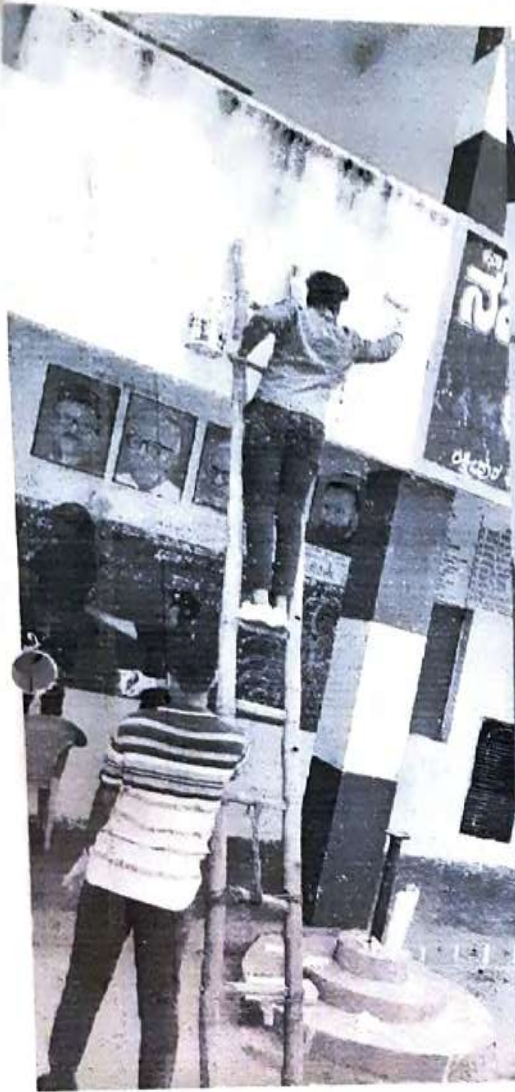
5: White wash before painting the wall
