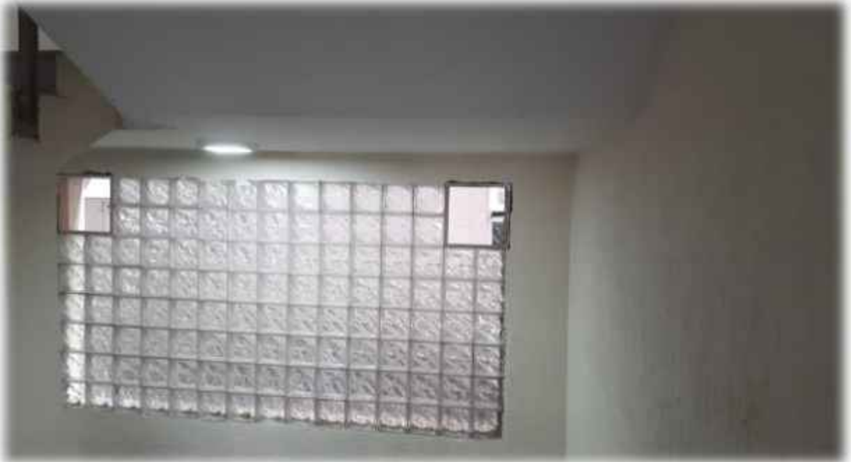
Ventilation on Duct
